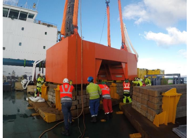
Figure 25 – 205Te ballast block
