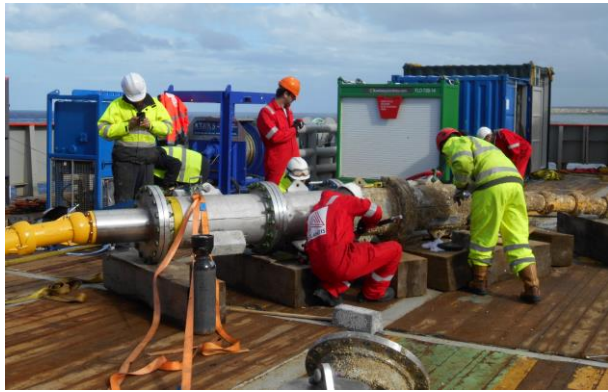
Figure 13 – Dry-mate connected on deck
