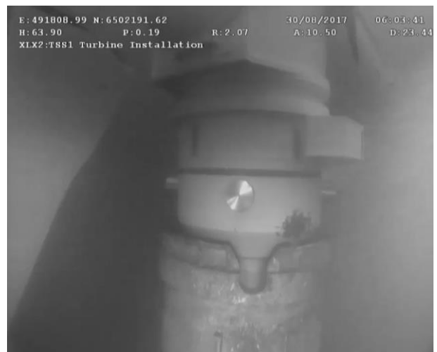
Figure 16 – Turbine stab being landed onto the TSS
