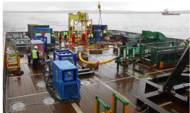
Figure 12 – Landing the export cable on deck
