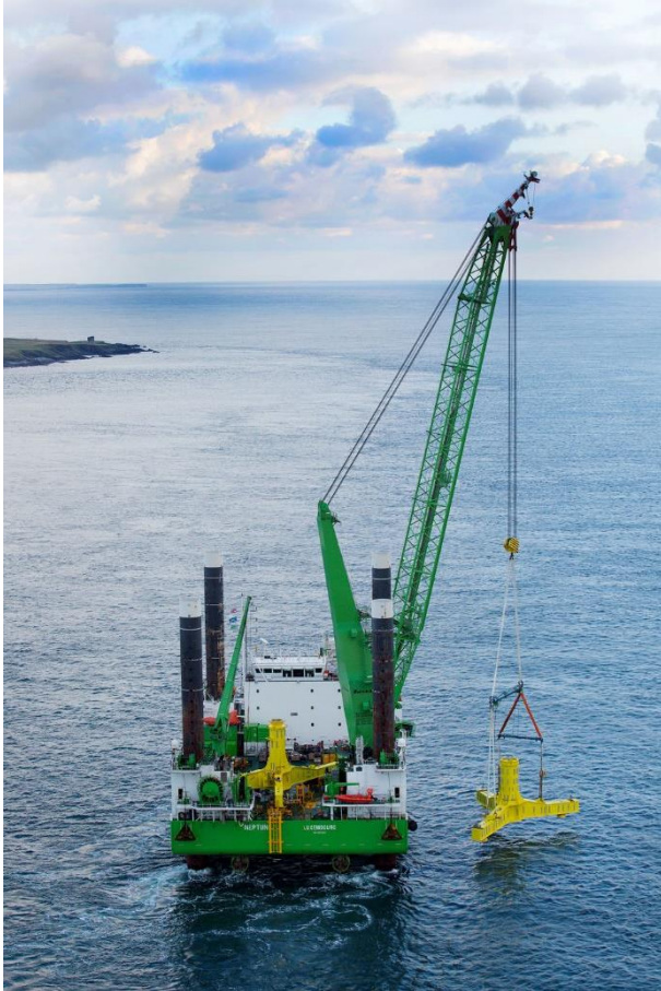
Figure 24 – TSS being installed in slack tide
