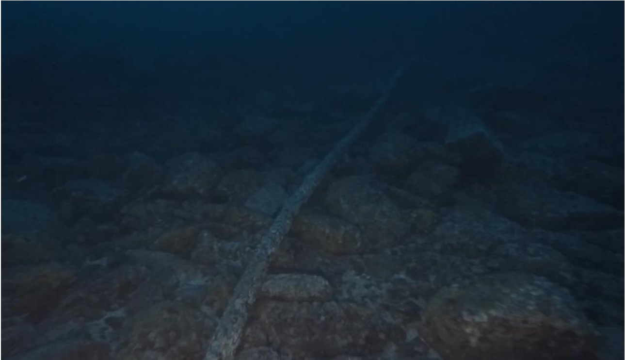
Figure 22 – MeyGen export cable laid on exposed bedrock
