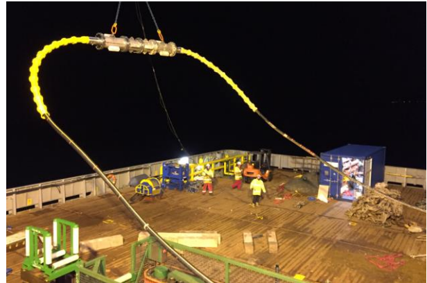
Figure 14 – Dry-mate being handled for deployment
