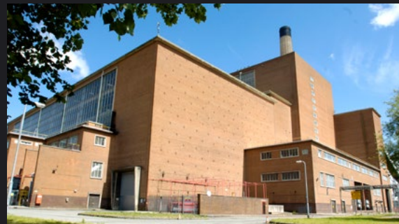
Uskmouth Power Station
