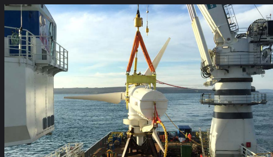
AHH 1.5 MW turbine lift
