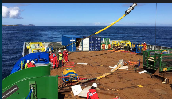
Andritz dry mate cable connection
