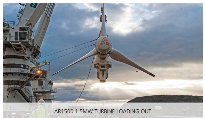
ARL NACELLE INSTALLATION TOOL BEING PREPARED TO LOAD THE AR1500 1.5MW TURBINE
